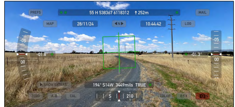
Photo Point 23. Looking at the existing well-maintained access road from TransGrids Wagga North Zone substation heading towards Byrnes Rd located west adjacent to the proposed WNBESS development site. (Hague, 2024)
