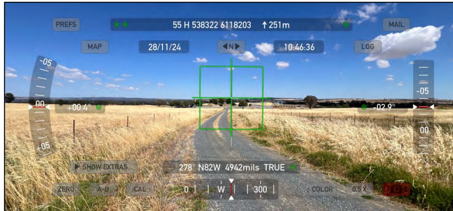
Photo Point 21. Looking at the existing well-maintained access road from the TransGrid Wagga North Zone substation heading towards Byrnes Rd. (Hague, 2024)
