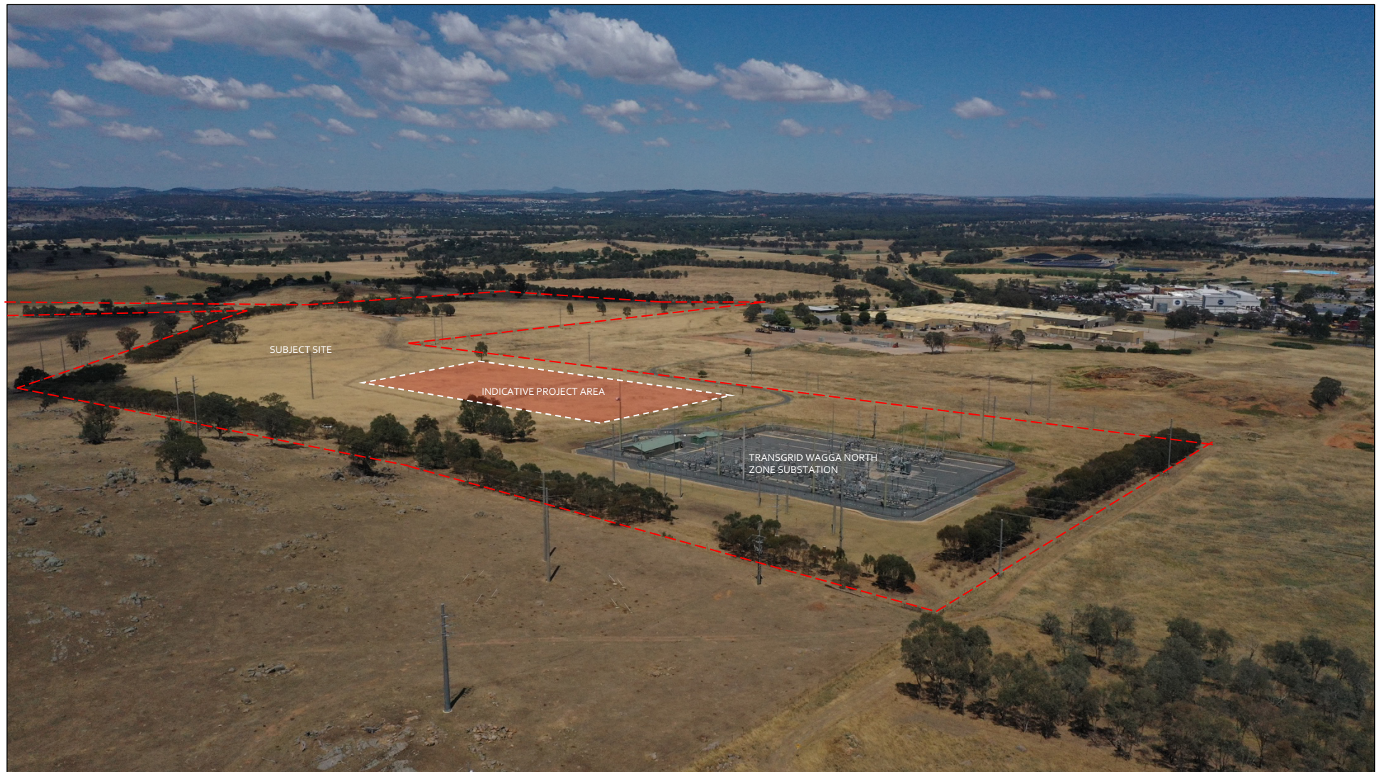
Photo Point A2. Looking southwest at the Subject Site and indicative Project Area showing the extent of surrounding hazard vegetation and existing development and the adjacent TransGrid Wagga North Zone Substation. (Hague, 2024)
