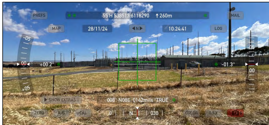
Photo point 6. Looking at the TransGrid Wagga North Zone Substation north of the proposed WNBESS Project Area. (Hague, 2024)
