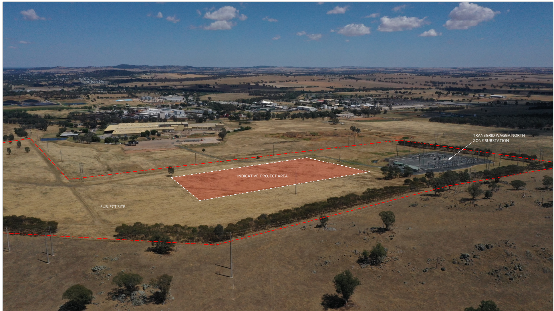
Photo Point A3. Looking northwest at the Subject Site and indicative Project Area showing the extent of surrounding hazard vegetation and existing development and the adjacent TransGrid Wagga North Zone Substation. (Hague, 2024)
