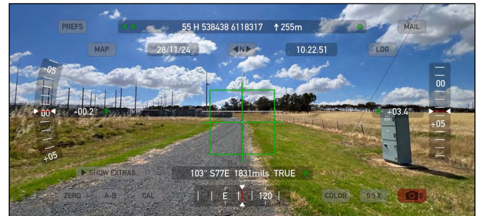
Photo point 24. Looking at the existing well-maintained access road and entrance point to TransGrids Wagga North Zone substation located north adjacent to the proposed WNBESS development site. (Hague, 2024)
