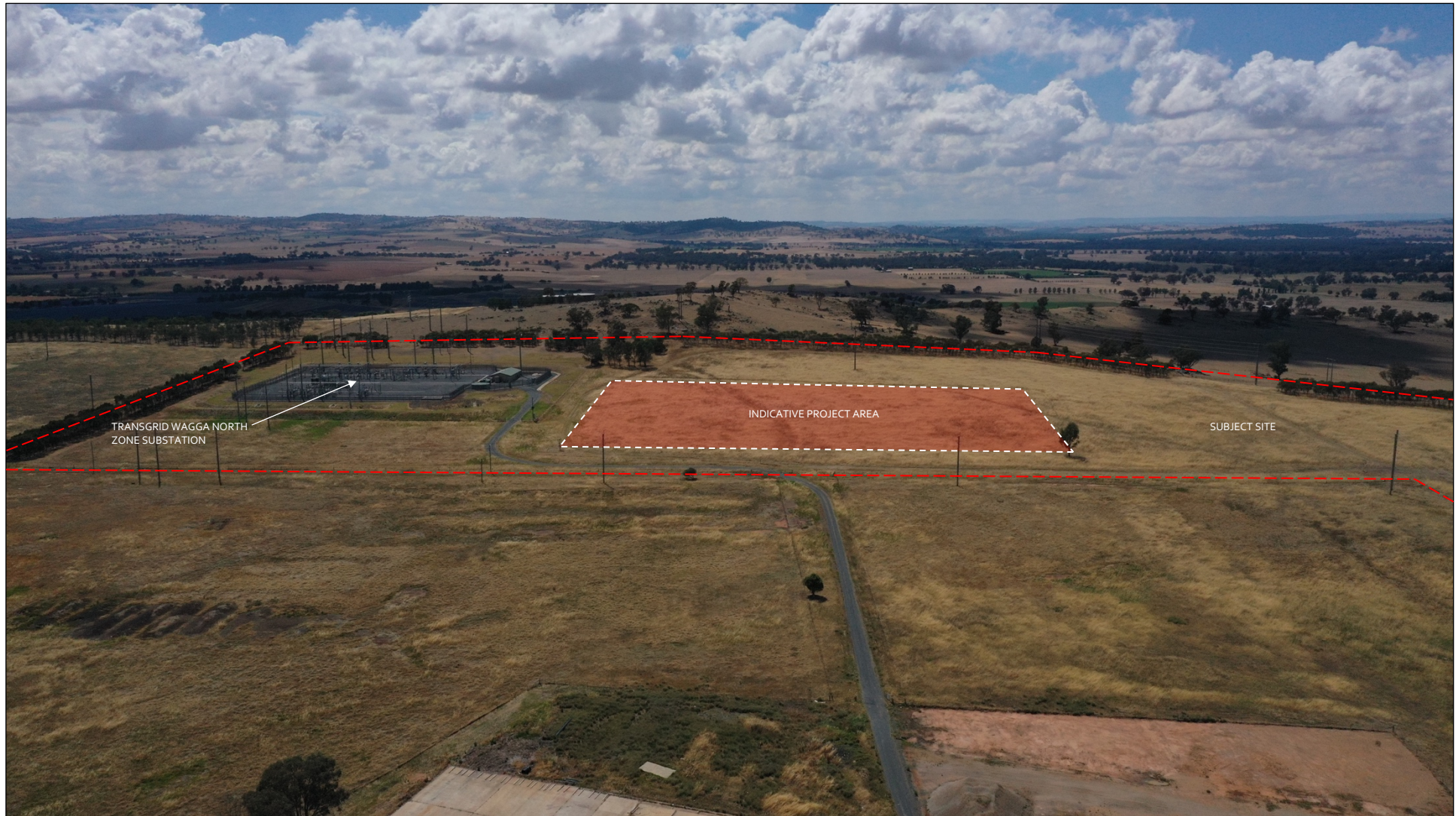
Photo Point A5. Looking west at the Subject Site and indicative Project Area showing the extent of surrounding hazard vegetation and the adjacent TransGrid Wagga North Zone Substation. (Hague, 2024)
