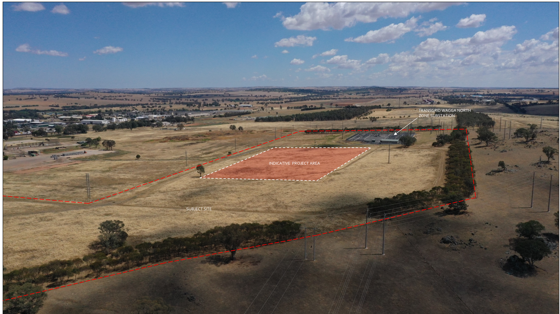
Photo Point A4. Looking north at the Subject Site and indicative Project Area showing the extent of surrounding hazard vegetation and existing development and the adjacent TransGrid Wagga North Zone Substation. (Hague, 2024)
